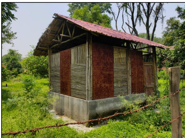
Fig 3: Hut made out of bamboo and bamboo laminates
